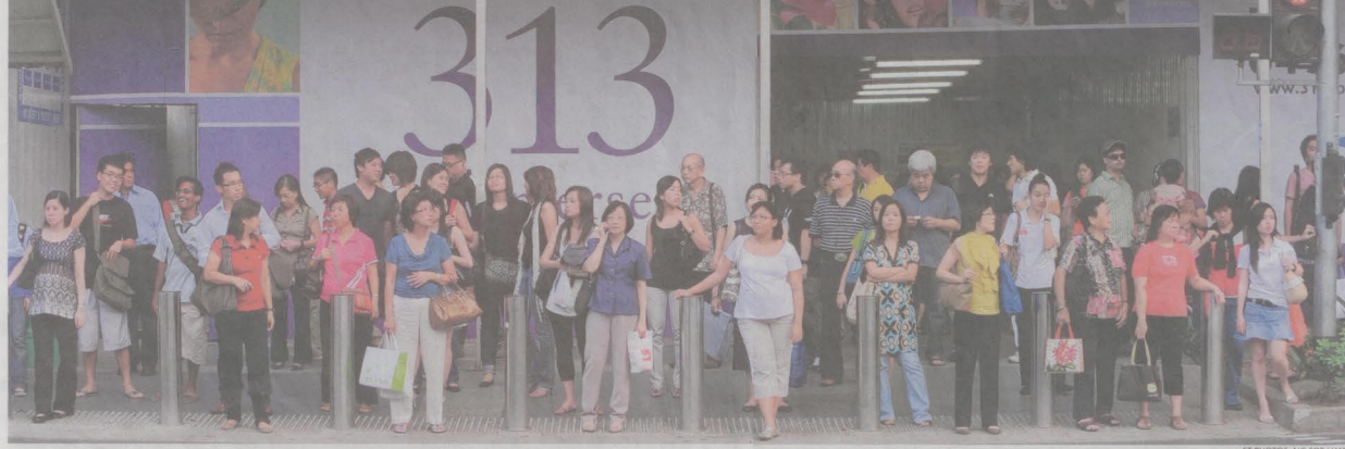
Pedestrians in front of the almost completed shopping mall 313@Somerset, which is due to open in November. Though shoppers say they prefer a wider variety of shops, experts say malls tend to bring in tried and tested brands.
